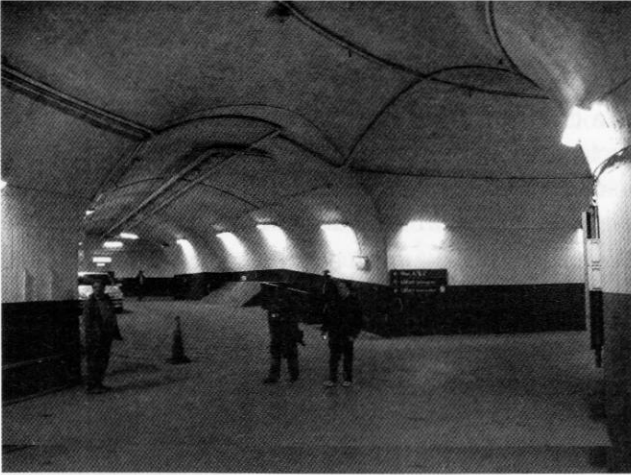
Spiral road allowing cars to descend to the three floors of the shelter. Photo Clive Penfold
